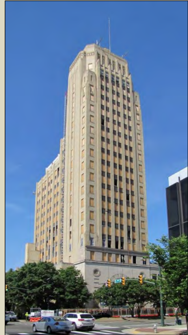
The former Central National Bank is an example of an Art Deco skyscraper. Designed by New York architect John Eberson with the local firm of Carneal, Johnston and Wright serving as consultants. 219 E. Broad St., Richmond, VA (1929-30) (photo by Chris Novelli)
