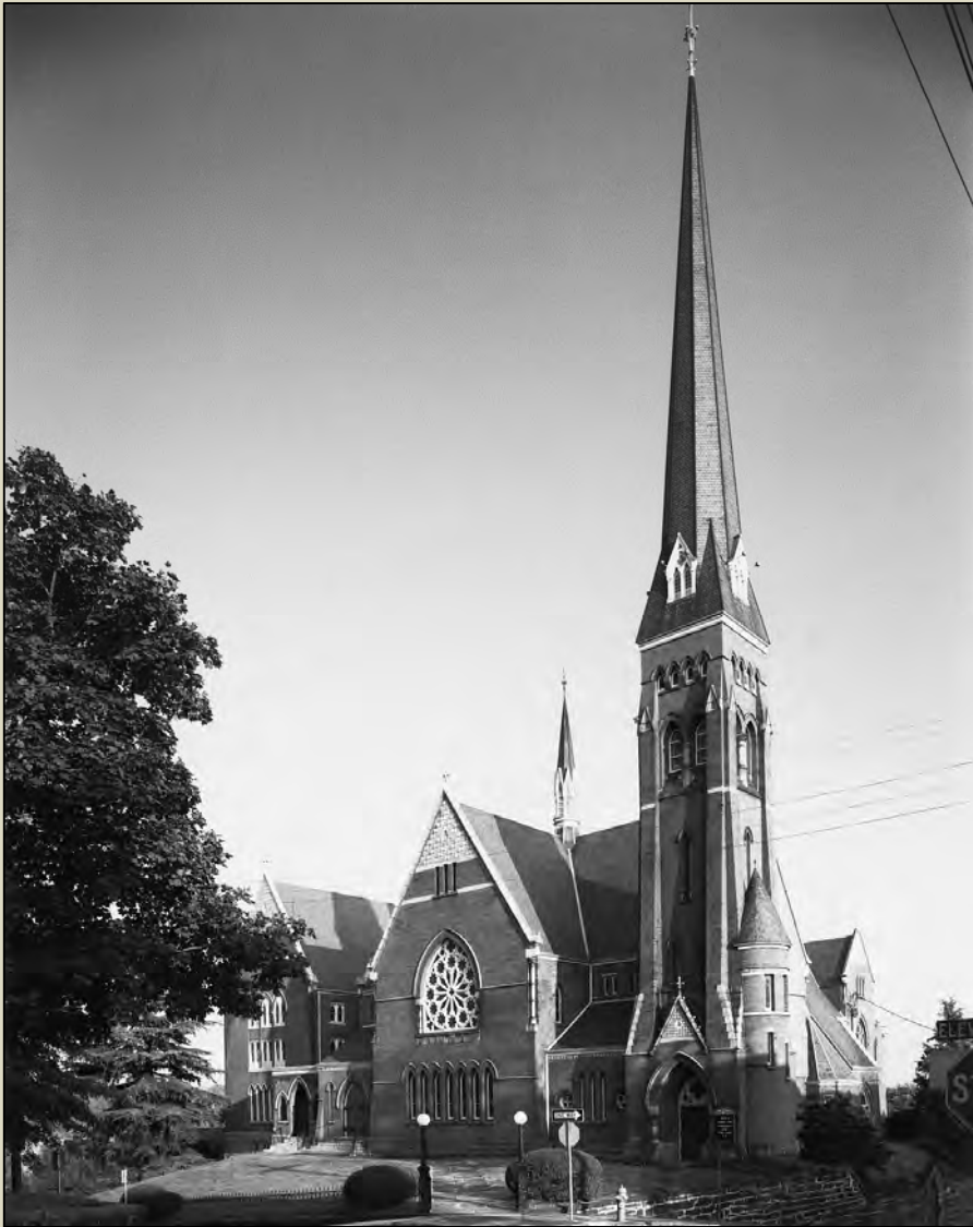
Designed by John R. Thomas, the First Baptist Church was built in 1886. Lynchburg, VA (photo from DHR)
