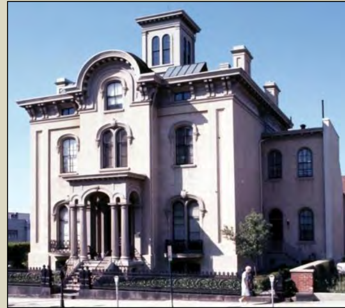
Bolling-Haxall House, Richmond, VA (1858) (photo from DHR)
