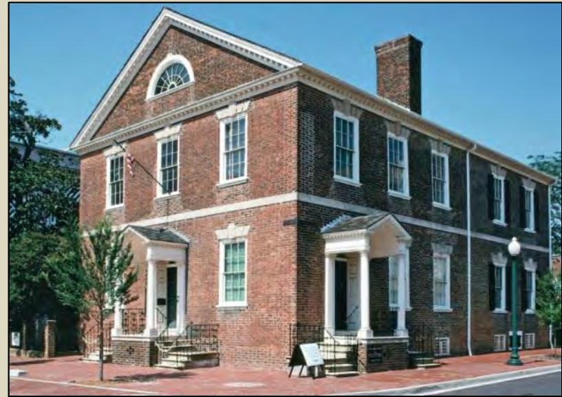
Moses Myers House, 331 N. Bank St., Norfolk, VA (c. 1792) (photo: Calder Loth)
