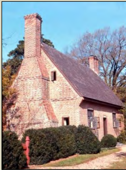
Thoroughgood House, Virginia Beach, VA (c. 1720) (photo from DHR)
