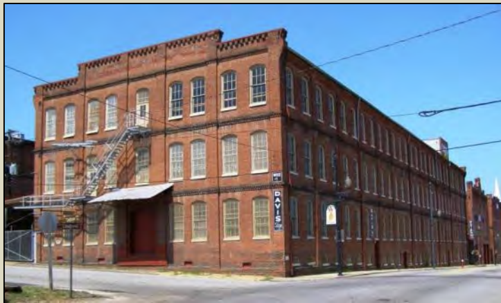
A warehouse in the Danville Tobacco Warehouse and Residential Historic District, Danville, VA (photo from DHR)
