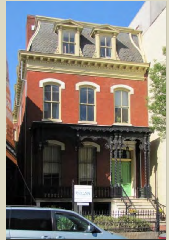
The Winston House at 103 E. Grace St. in Richmond has an S-curved mansard roof and pedimented dormers. (1874) (photo by Chris Novelli)
