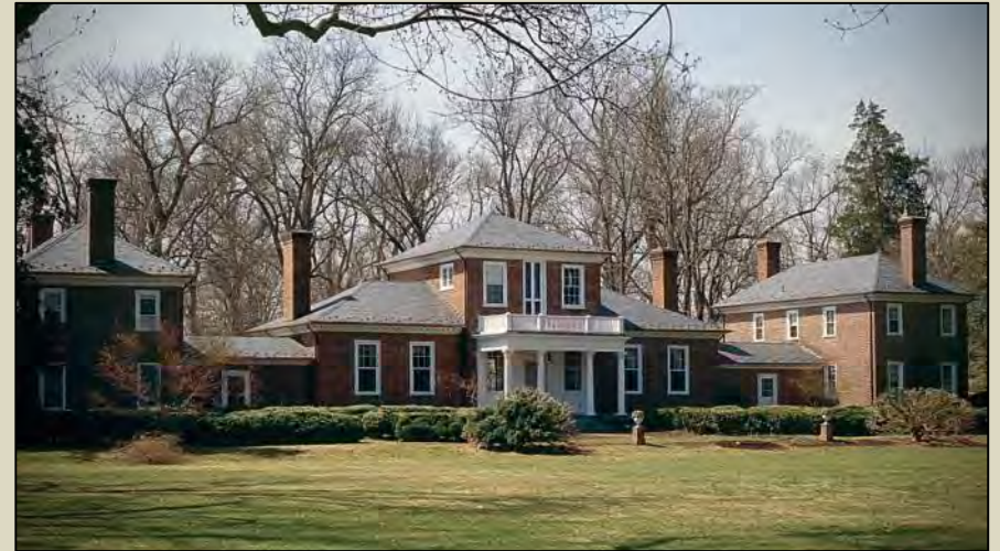
Brandon in Prince George County is a seven-part Palladian house. (Wings: c. 1750; central block: after 1795) (photo by Calder Loth)
