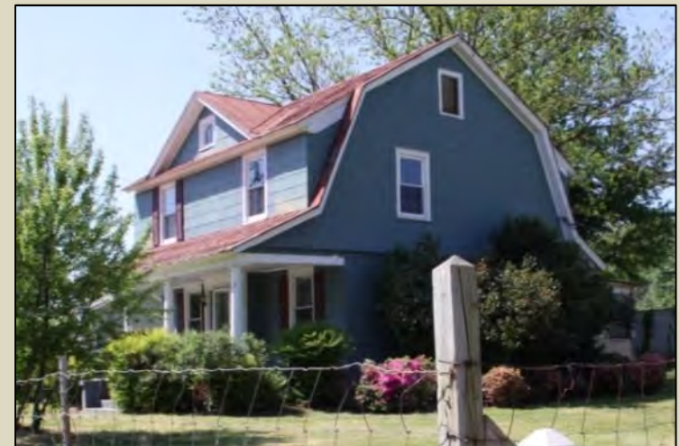
Side-gambrel house with a continuous shed dormer in Colonial Heights, VA (photo from DHR)
