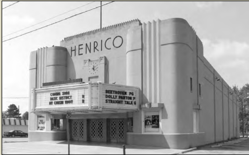
Henrico Theater, Highland Springs, VA (1938) (photos from DHR)
