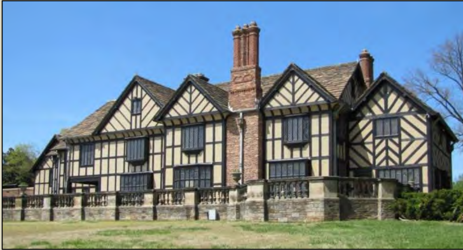
Agecroft Hall is a 16 th -century Tudor manor house from England which was disassembled, shipped, and rebuilt in Richmond in 1926-1928. (photo: C. Novelli)
