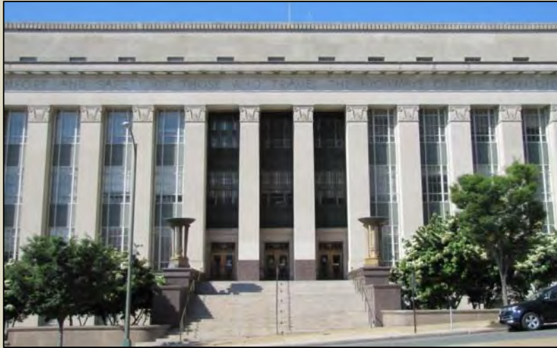
The Virginia Department of Highways Building, architects Carneal, Johnston and Wright, Richmond, VA (1939) (photo by Chris Novelli)
