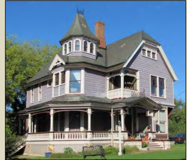
Superintendent's House, Hollywood Cemetery, Richmond, VA (1895) (photo by Chris Novelli)
