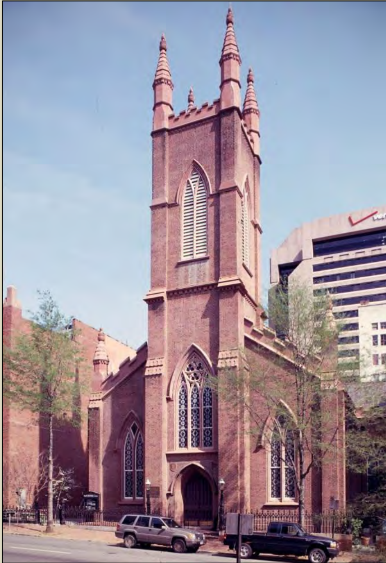
Second Presbyterian Church, Richmond, VA (1848) (photo: Calder Loth)
