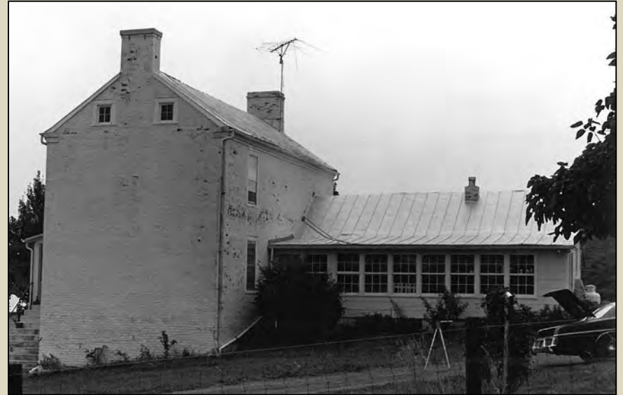
The Augusta County Poorhouse features an L-plan form. Augusta County, VA (photo from DHR)
