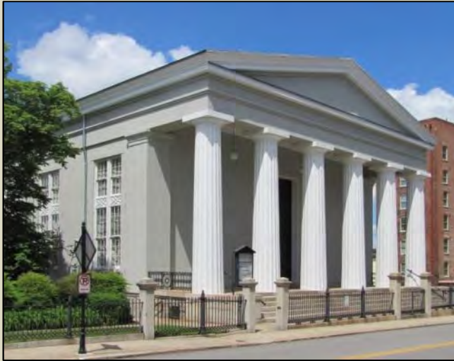
Tabb Street Presbyterian Church, Petersburg, VA, Thomas U. Walter, architect (1843) (photo by Chris Novelli)
