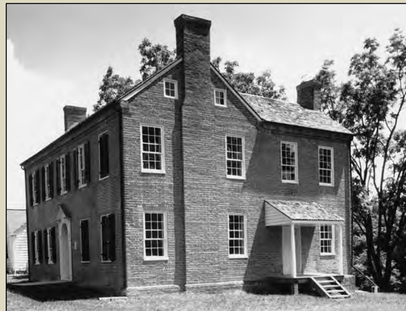
The Miller-Kite House is a brick I-House first built in 1829 with a rear lean-to added in 1848 (pictured). Elkton, VA (photo from DHR)
