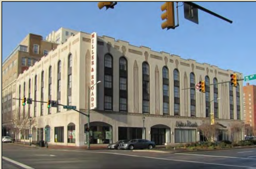
Former Miller & Rhoads Department Store, 517 E. Broad St., Richmond, VA (c. 1935) (photo by Chris Novelli)
