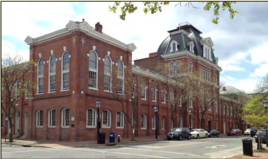
Alexandria City Hall, Alexandria, VA (1871) (photo by Geo-Technology Associates, Inc.)
