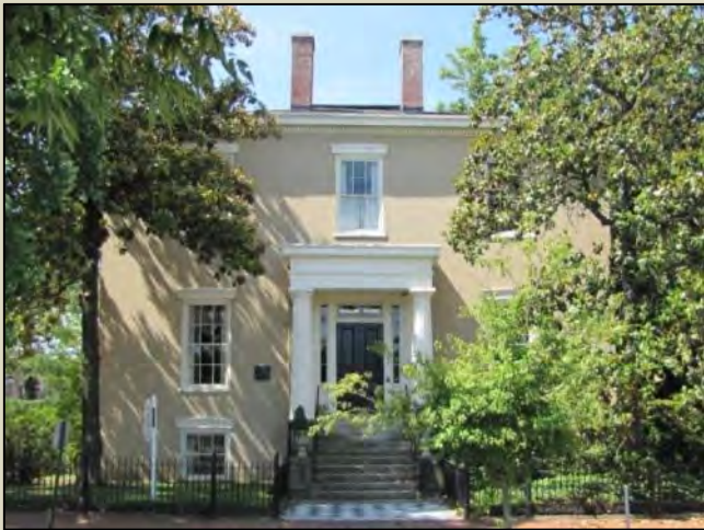
Ellen Glasgow House, 1 W. Main St., Richmond, VA (1841) (photo by Chris Novelli)
