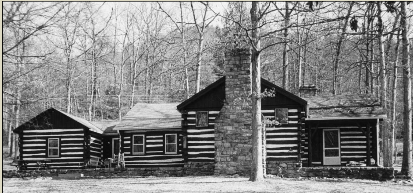
This building in Douthat State Park was built by the C.C.C. during the Great Depression. Millboro, VA (photo from DHR)
