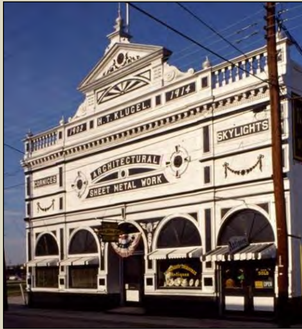
H. T. Klugel Architectural Sheet Metal Work building, 135 Atlantic Street, Emporia, VA (1914) (photo from DHR)
