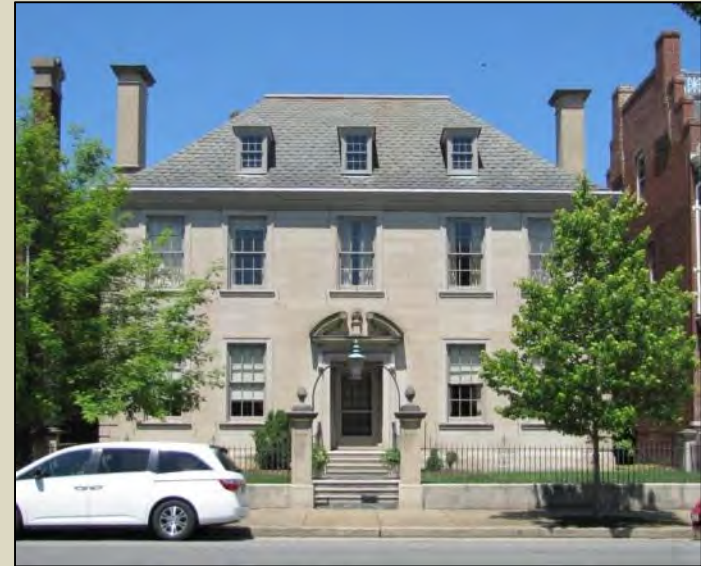
McGuire House, Monument Ave., Richmond (photo: Chris Novelli)
