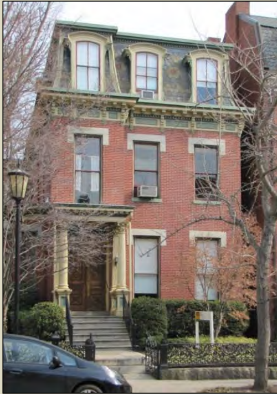
The Gunn-Bird House at 820 W. Franklin St. in Richmond has a concave mansard roof and segmental dormers. (1886) (photo by Chris Novelli)
