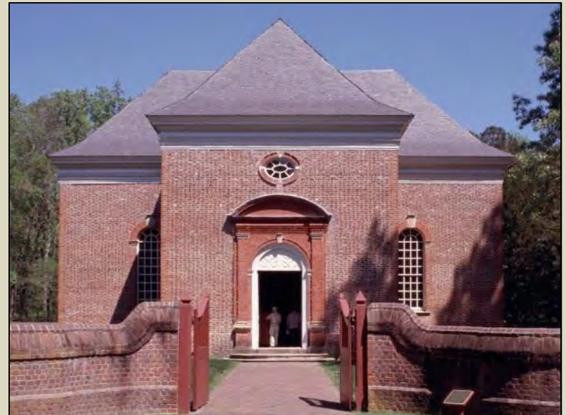
Christ Episcopal Church, Lancaster Co., VA (1735) (photo by Calder Loth)
