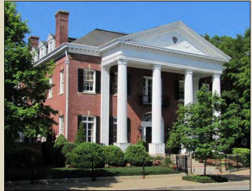
The Blair House, 2327 Monument Avenue, Richmond, VA (1913) (photo by Chris Novelli)
